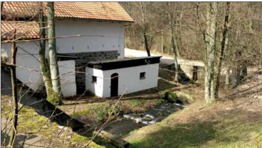
Fig. 8. A view of the seventh position, and the area between positions 6 and 7 – March 2016 (photo: Parszuto)
